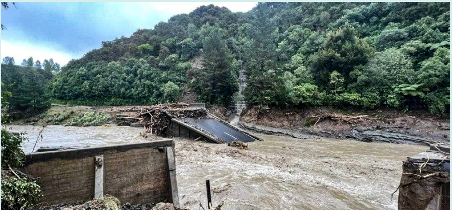
Collapse of Waikare Bridge after floods (Waka Kotahi)
